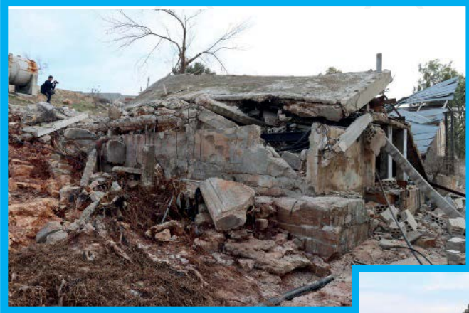
After the assault, the 2nd water station will be built.
