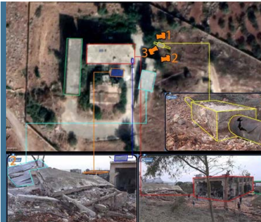
Image: Satellite image of Al-Arshani Water Pumping Station and site images after the attack. (Orange icons in the shape of cameras denote the locations where the photographs were taken). [Syrian Archive]
